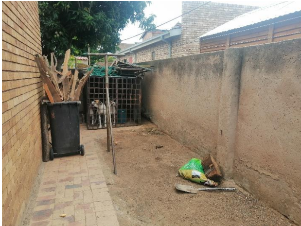
Fig 1.5 shows the clearing of timber from the ground.
