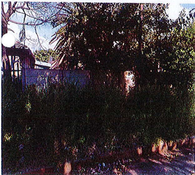
Image 2 and 3 Unkept, untidy and unsuitable living condition reason to believe abandoned.
