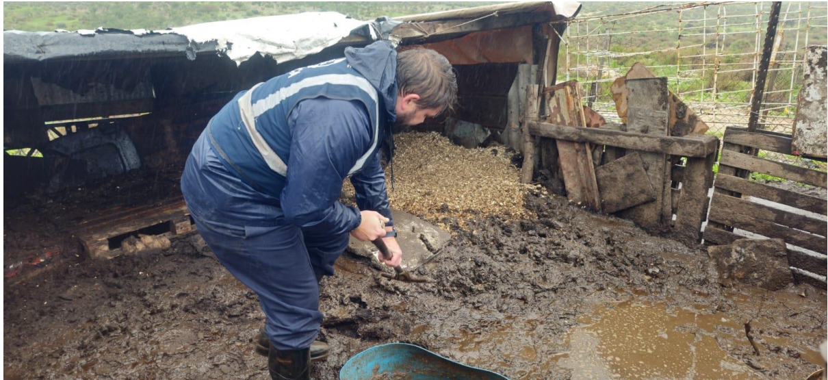
Photo 33: Inspector White digging drainage for Ockie Prins pig enclosure.
