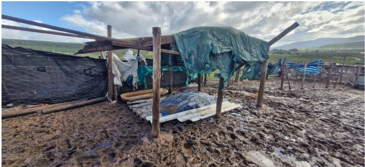
Photo 32: After shelter was fixed.
