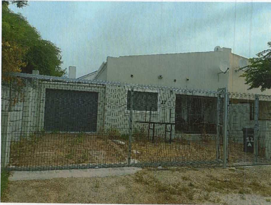
Picture 2: Property from the front.
