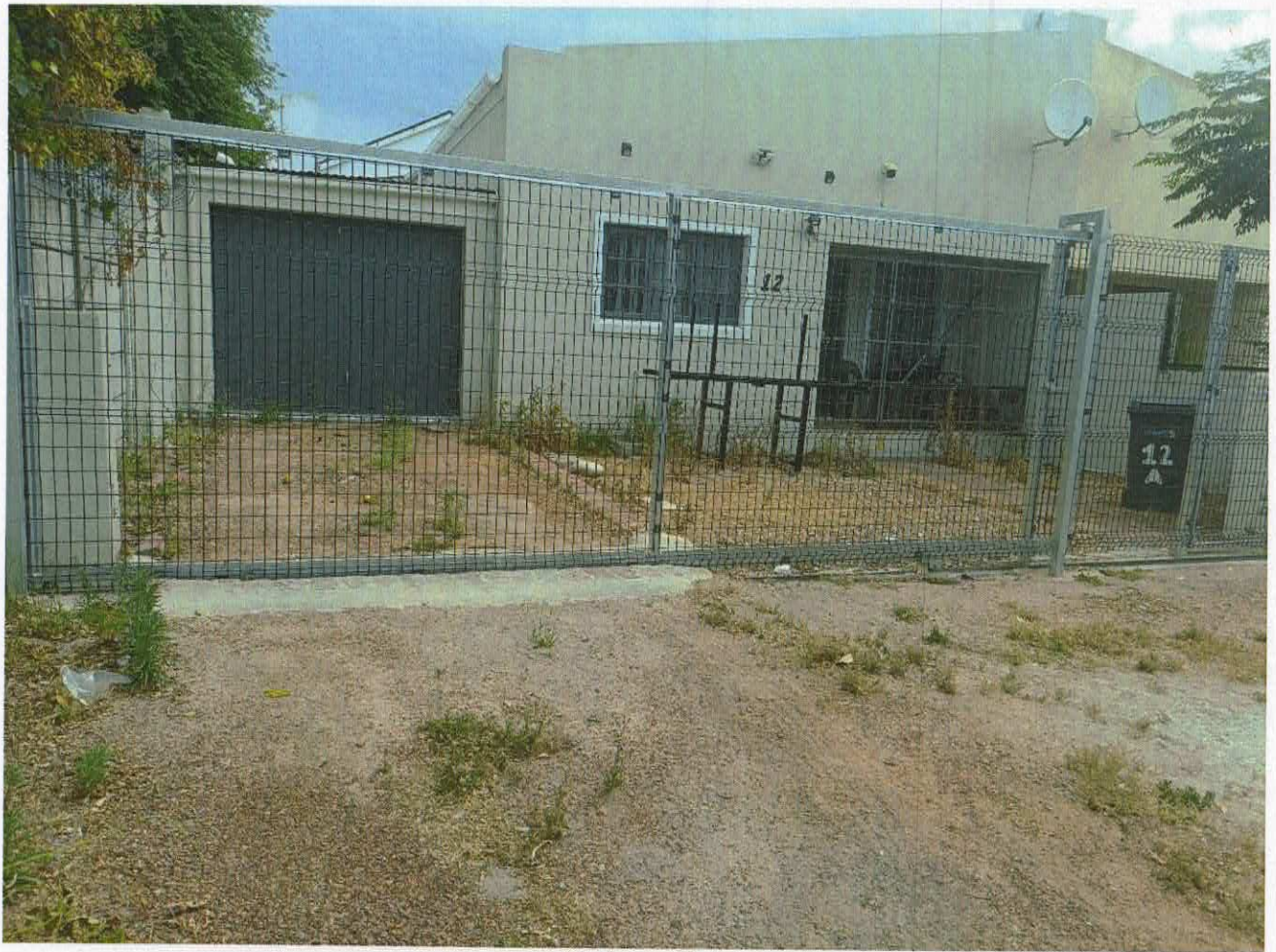
Picture 7: Property seen from the front yard.
