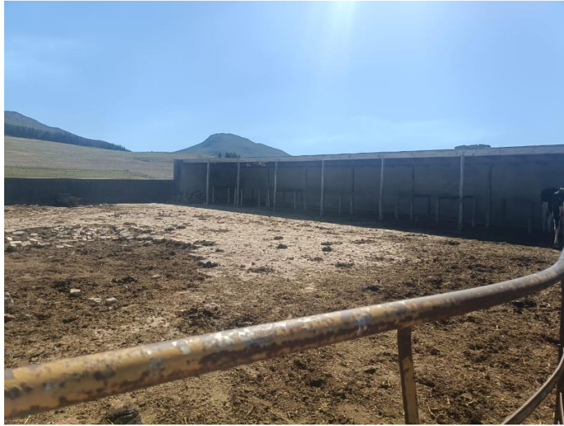
Figure 10: One of the outside camps with hazardous material and excess faeces seen with cattle inside.
