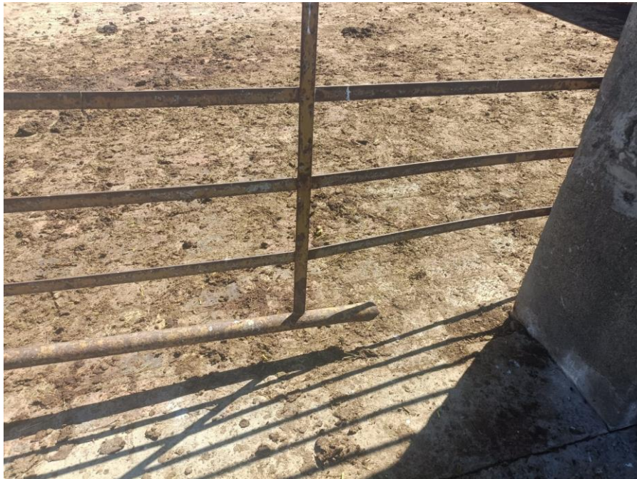
Figure 11: Broken, rusted gate with a sharp edge at one of the outside camps holding calves.
