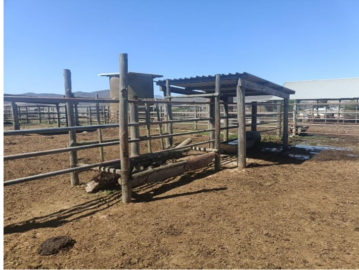
Figure 9: Old, unused, rusted trough seen in outside night cattle enclosure.
