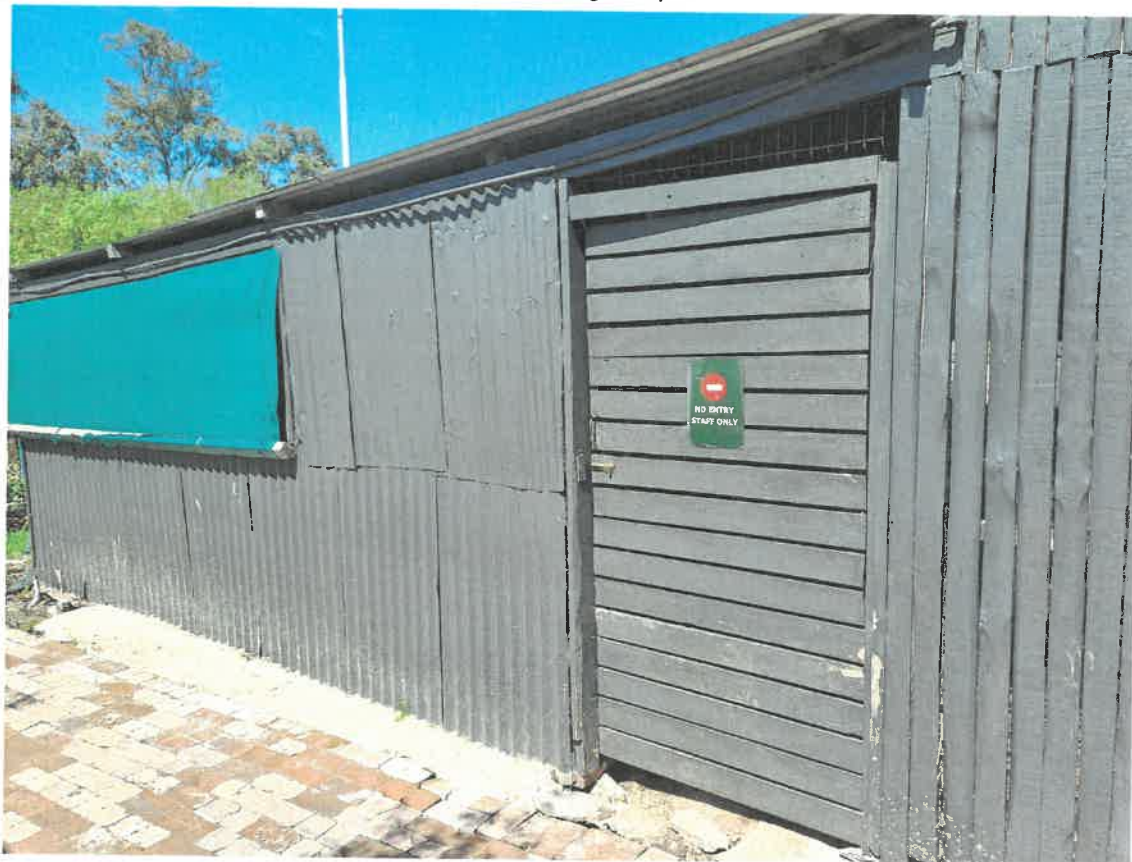
Photograph 03 – Depicting a close up of the shed referred to and seen in Photograph 02.
