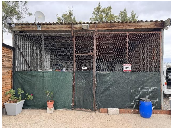
From the outside of Food storeroom (quarantine area)
