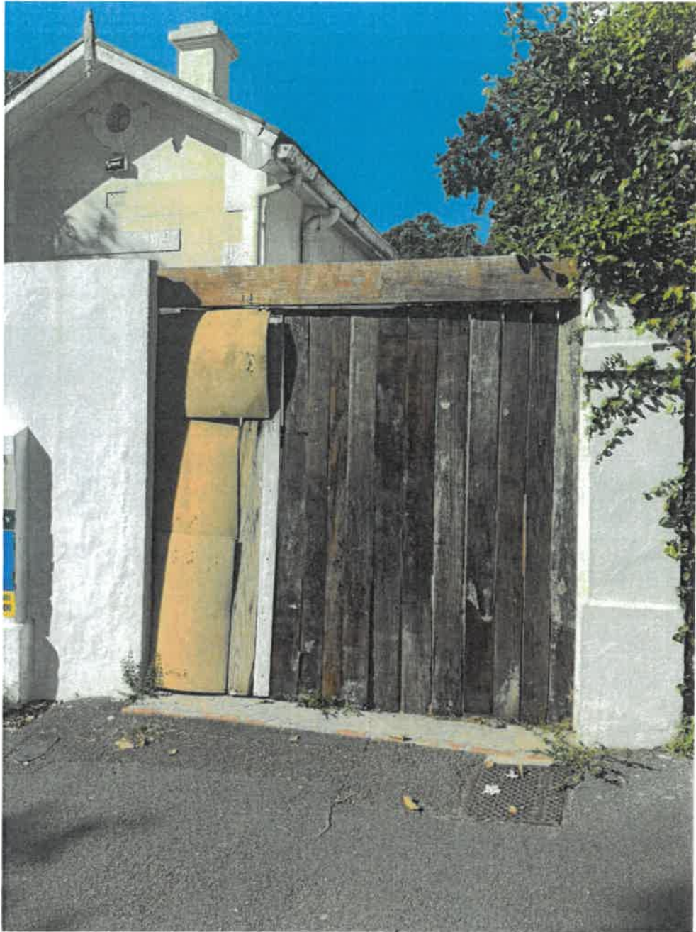
Figure 3 - Main access point into the property
