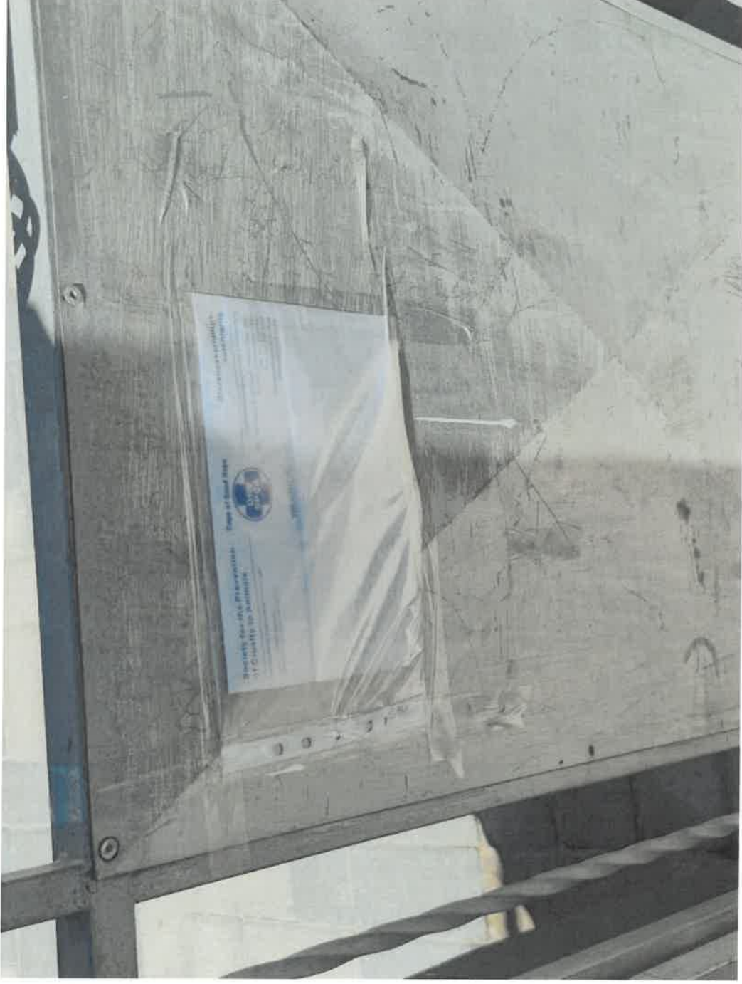
Photo 7 - Warning notice affixed to the gate
